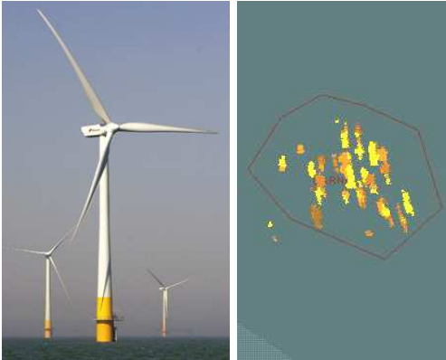
Figure 1 The moving blades of a wind turbine (left) can cause interference to Air Traffic Control Radar (right).
