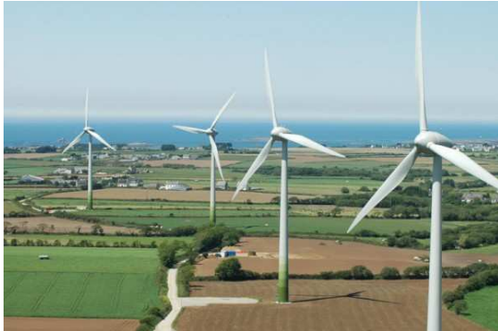
Figure 1 The moving blades of a wind turbine can cause interference to Air Traffic Control Radar.
