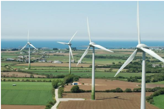
The moving blades of a wind turbine can cause interference to Air Traffic Control Radar.
